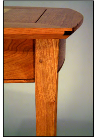
DETAIL Pinned mortise & tenon joinery splined miters curving aprons
